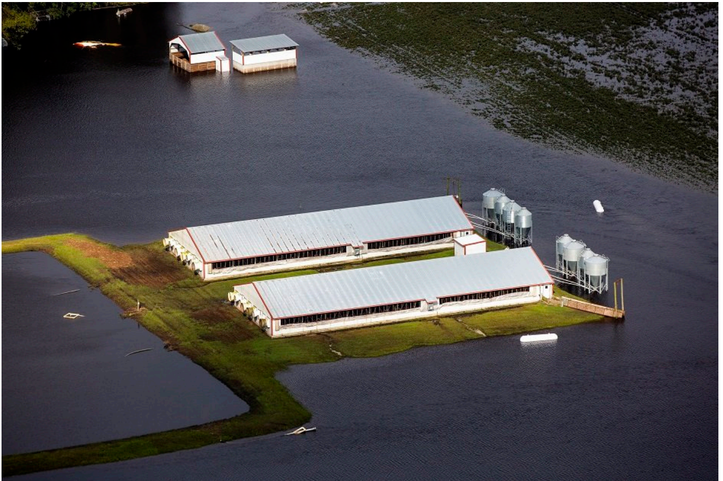
Hog Farm Flooded by Hurricane Florence
